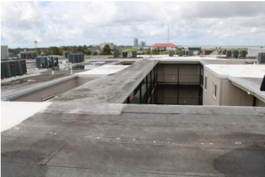
Photograph 30 - Rooftop from east edge – Looking west over open area below
