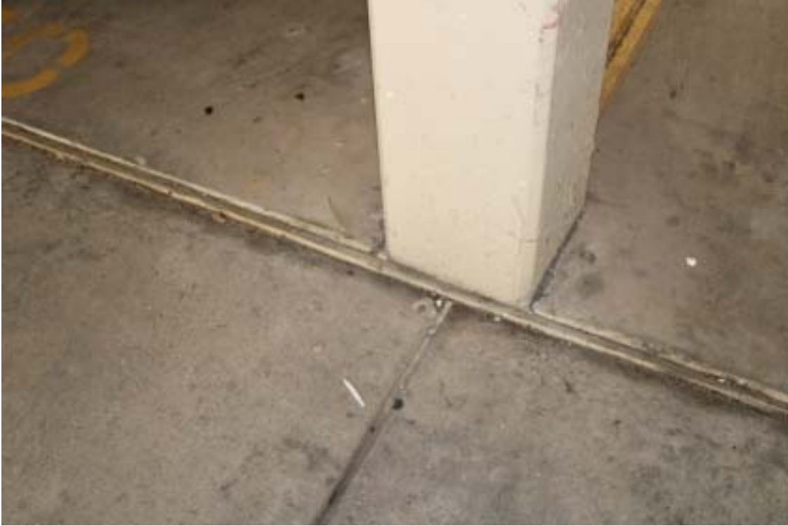
Photograph 51 - Concrete column below precast elements – Note typical base
