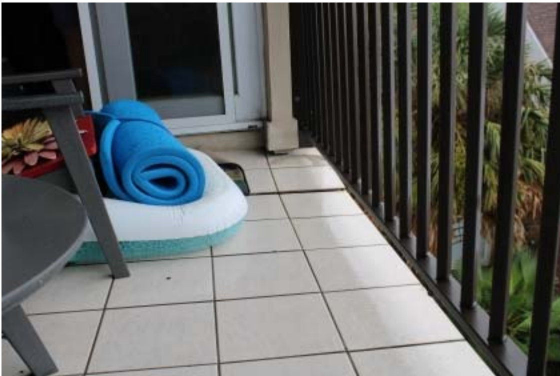
Photograph 64 - West side gallery floor – Tile over concrete topping
