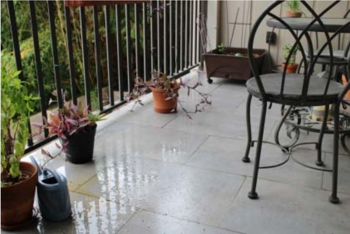
Photograph 67 - West side gallery floor – Tile over concrete topping
