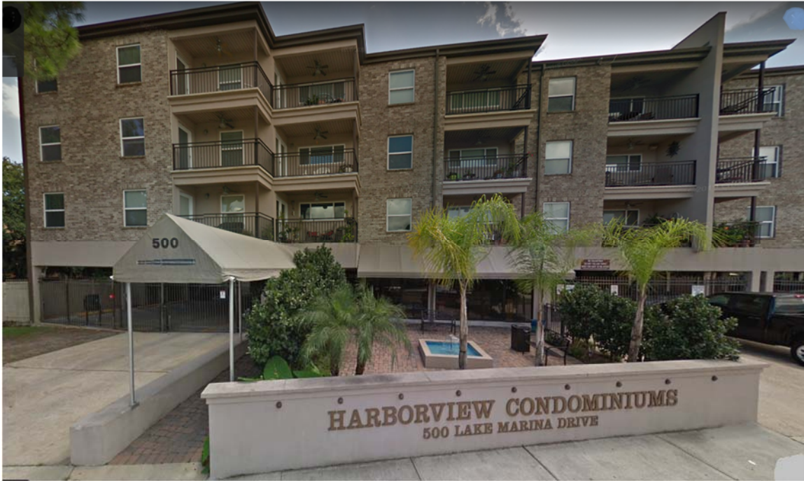
Photograph 1 - Front (north) elevation of building – 1 of 2
