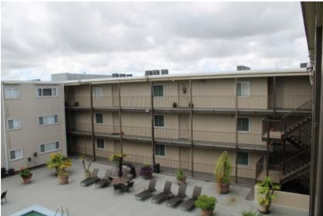
Photograph 12 - Interior upper hallway galleries – west side of pool area
