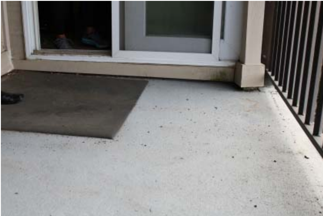
Photograph 60 - West side gallery floor – Concrete topping
