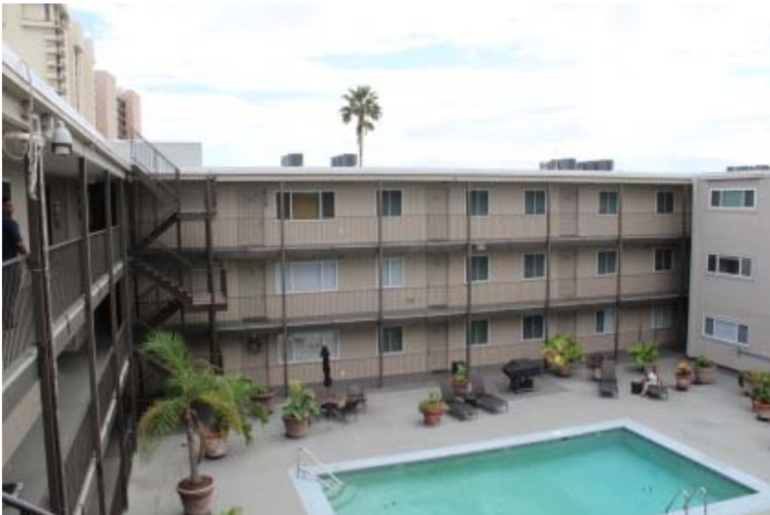
Photograph 14 - Interior upper hallway galleries – North and east sides of pool area
