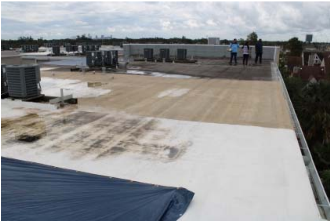
Photograph 22 - Rooftop from west edge – Looking south – Note varying roof colors
