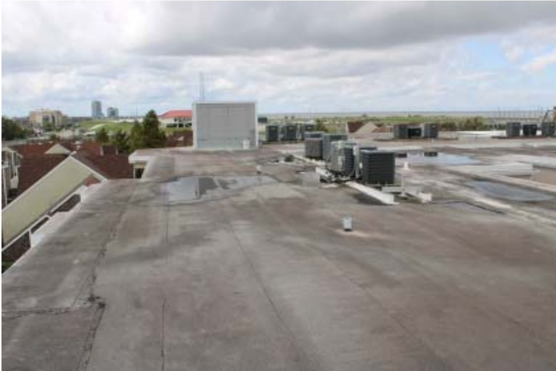
Photograph 27 - Rooftop from south edge – Looking west
