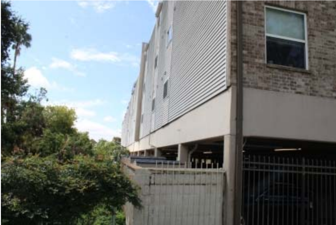
Photograph 11 - Northeast corner and east side of building
