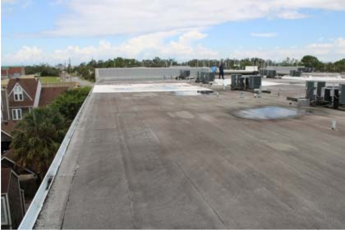
Photograph 25 - Rooftop from west edge – Looking north – Note varying roof colors
