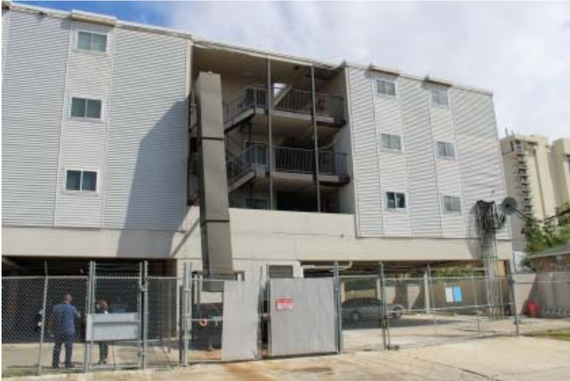
Photograph 9 - South side of building – 2 of 2
