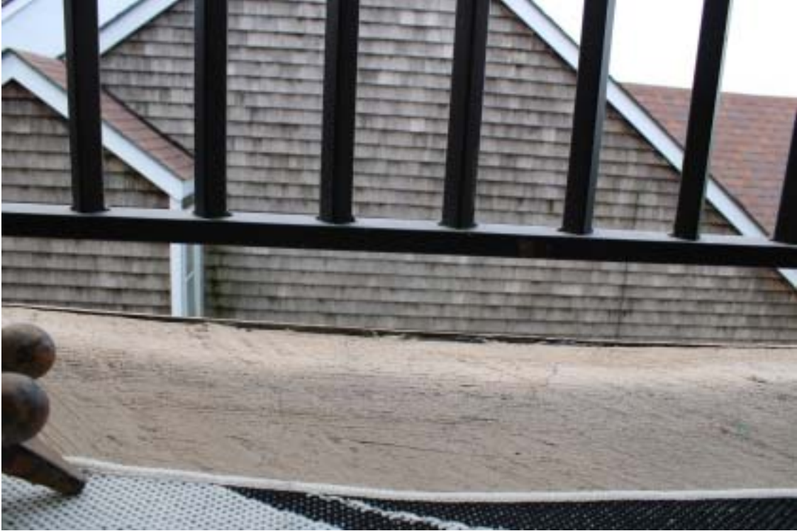
Photograph 61 - West side gallery floor – Concrete topping
