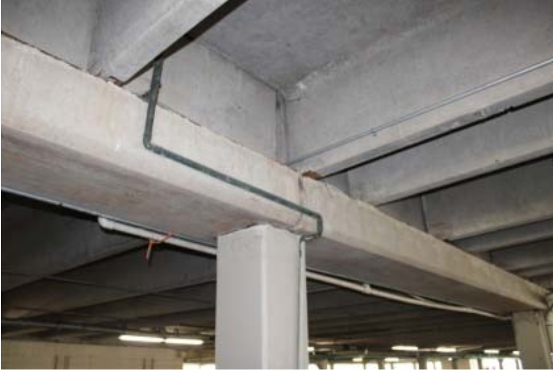
Photograph 39 - Concrete structure above parking level – Note precast elements
