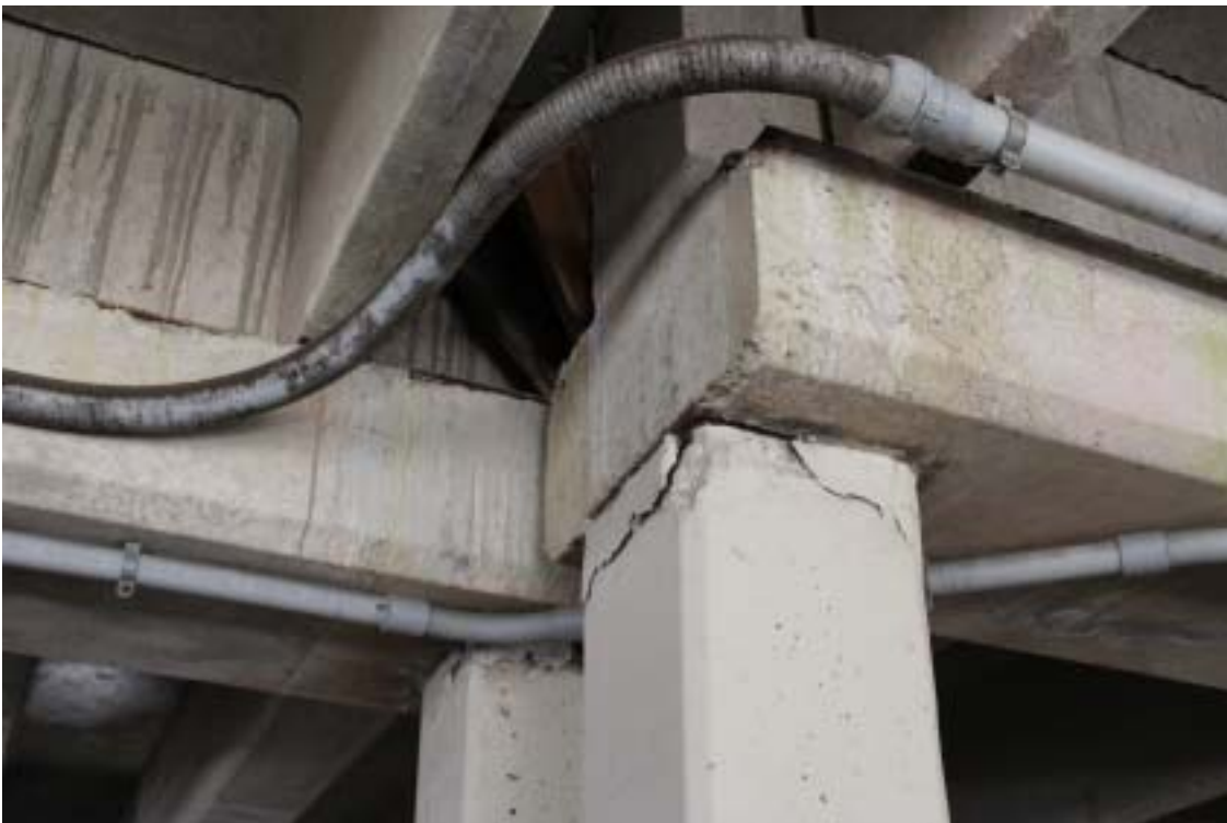
Photograph 36 - Concrete structure above parking level – Note precast elements
