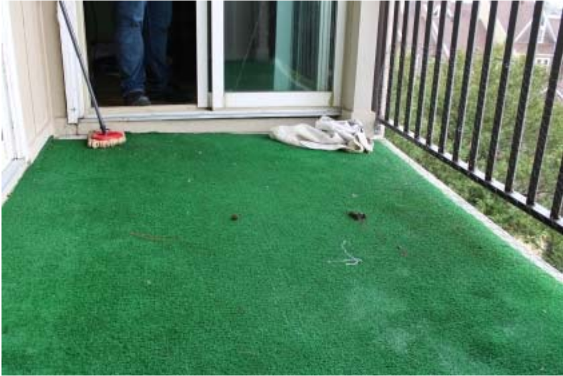
Photograph 65 - West side gallery floor – Outdoor carpet over deck
