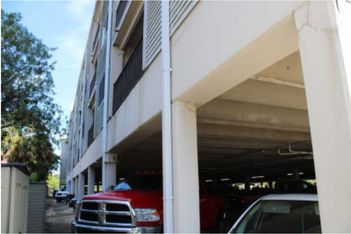
Photograph 7 - West side of building – From southwest corner
