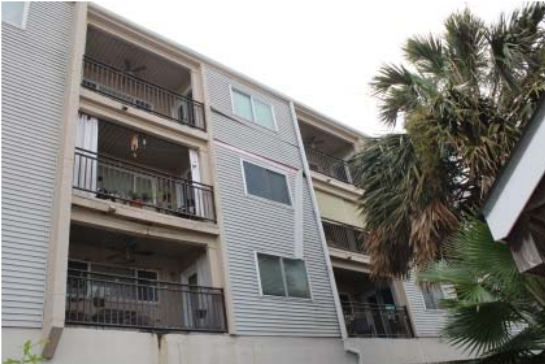
Photograph 6 - West side of building – Note upper side galleries – 3 of 3
