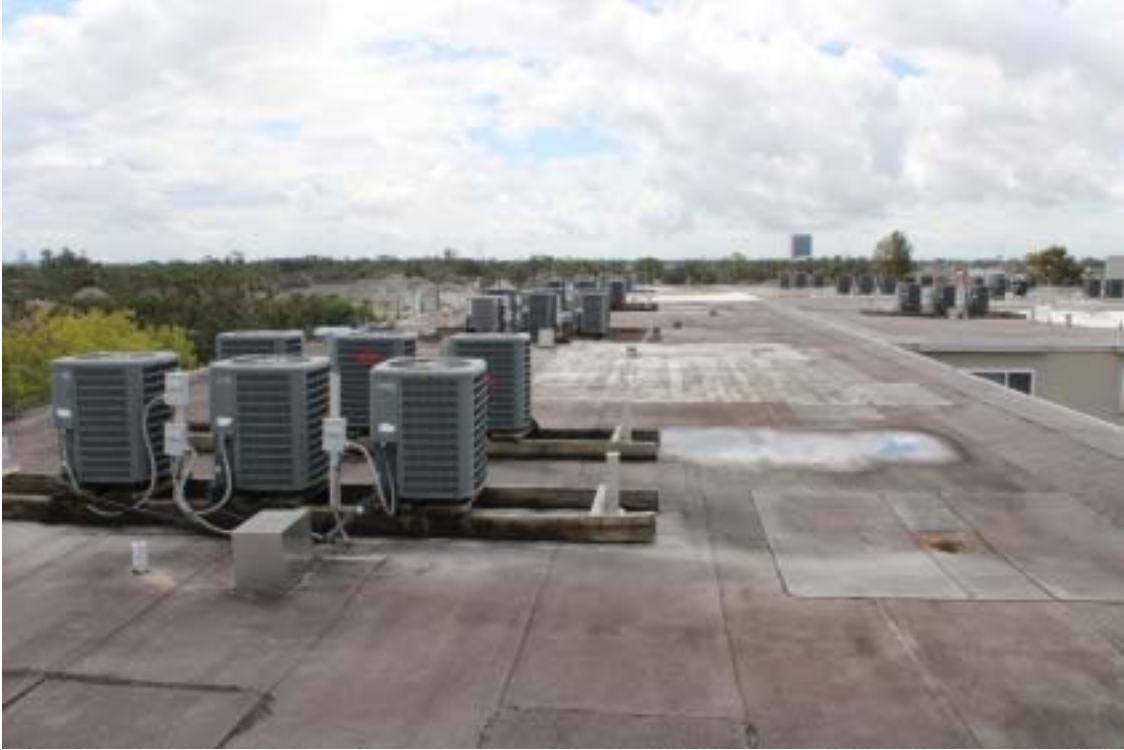
Photograph 31 - Rooftop from northeast corner – Looking south
