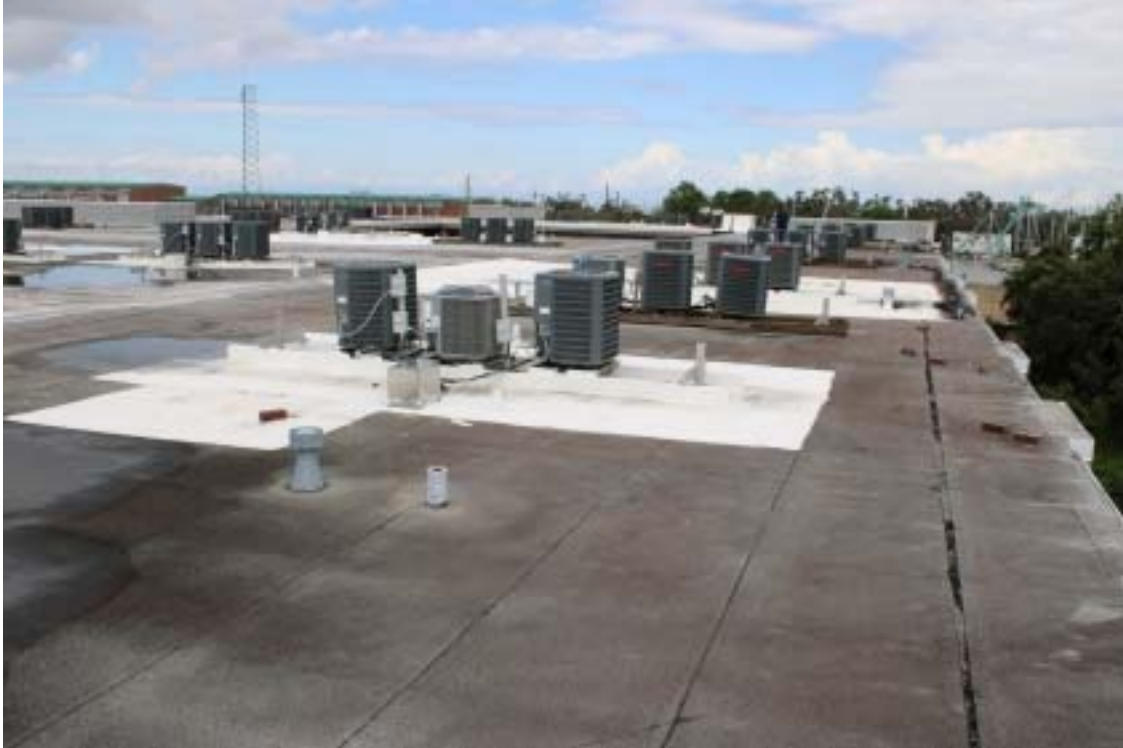
Photograph 29 - Rooftop from southeast corner – Looking north at light-colored roof areas
