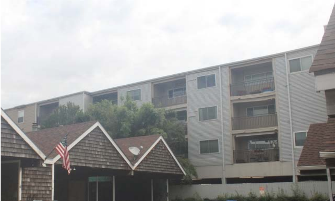
Photograph 5 - West side of building – Note upper side galleries – 2 of 3
