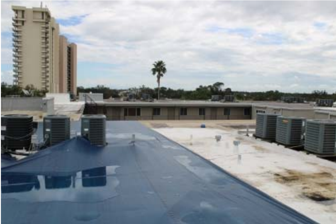
Photograph 21 - Rooftop from west edge – Looking east – Note blue tarp
