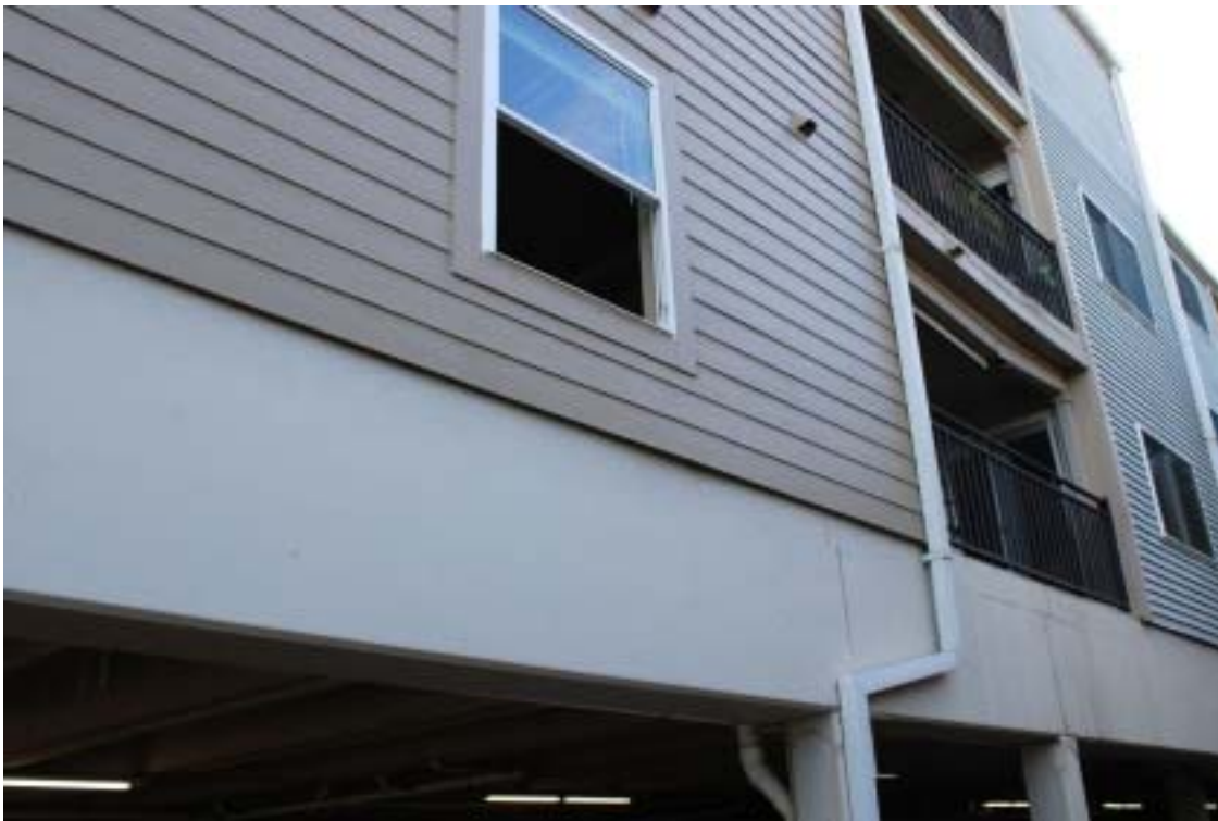
Photograph 4 - West side of building – Note upper side galleries – 1 of 3
