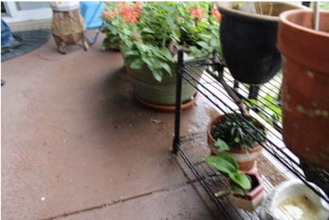
Photograph 66 - West side gallery floor – Concrete topping
