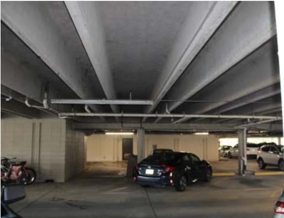
Photograph 32 - Concrete structure above parking level
