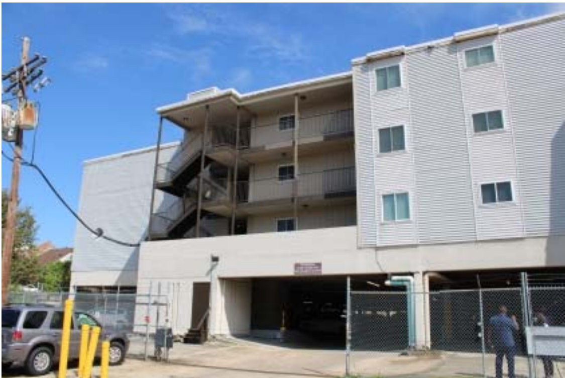
Photograph 8 - South side of building – 1 of 2
