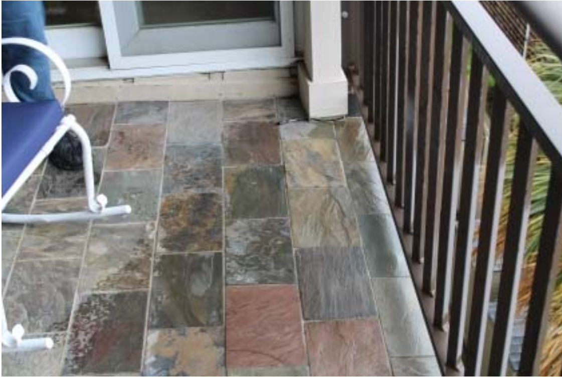
Photograph 63 - West side gallery floor – Tile over concrete topping
