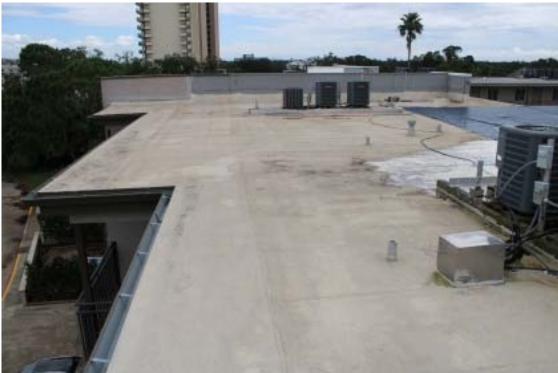
Photograph 18 - Rooftop from northwest corner – Note color and tarp to right
