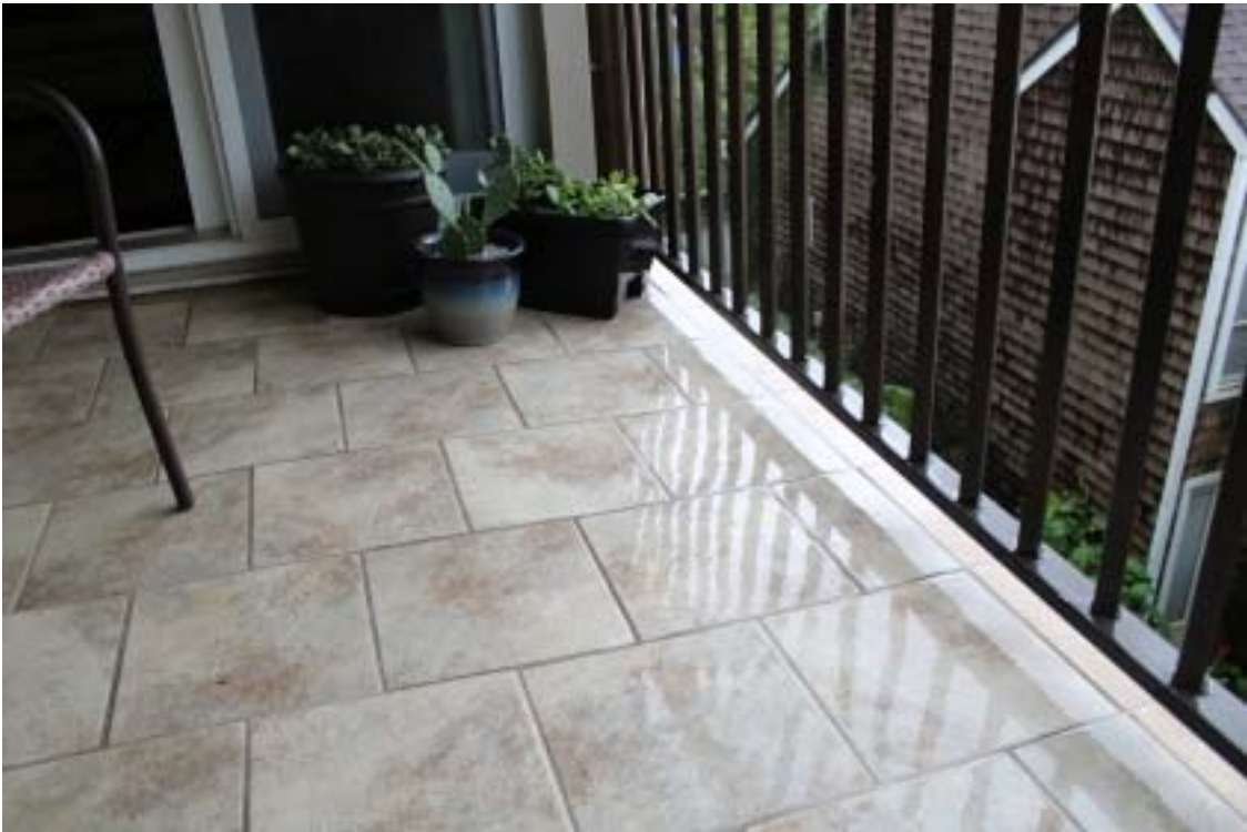
Photograph 62 - West side gallery floor – Tile over concrete topping
