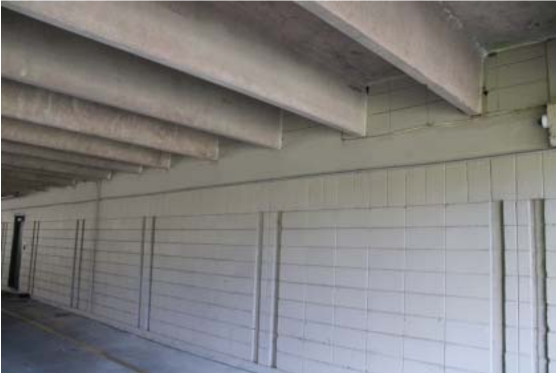
Photograph 33 - Concrete structure above parking level – Wall along office area
