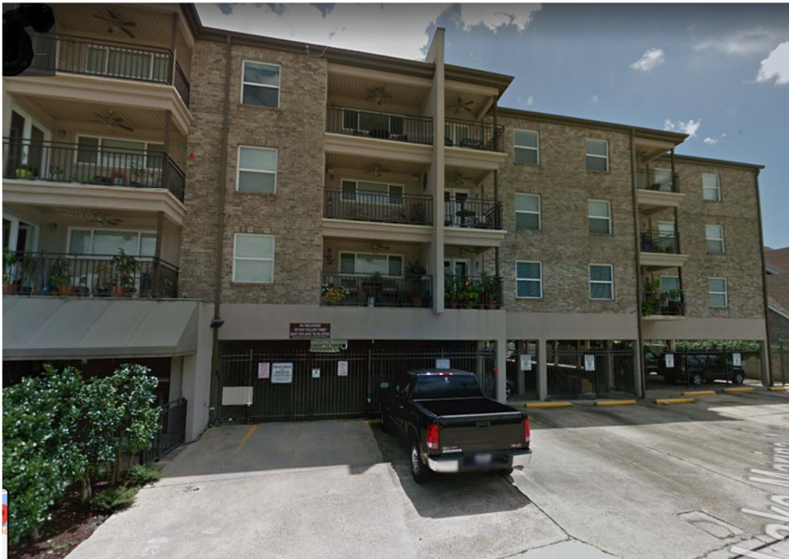
Photograph 2 - Front (north) elevation of building – 2 of 2
