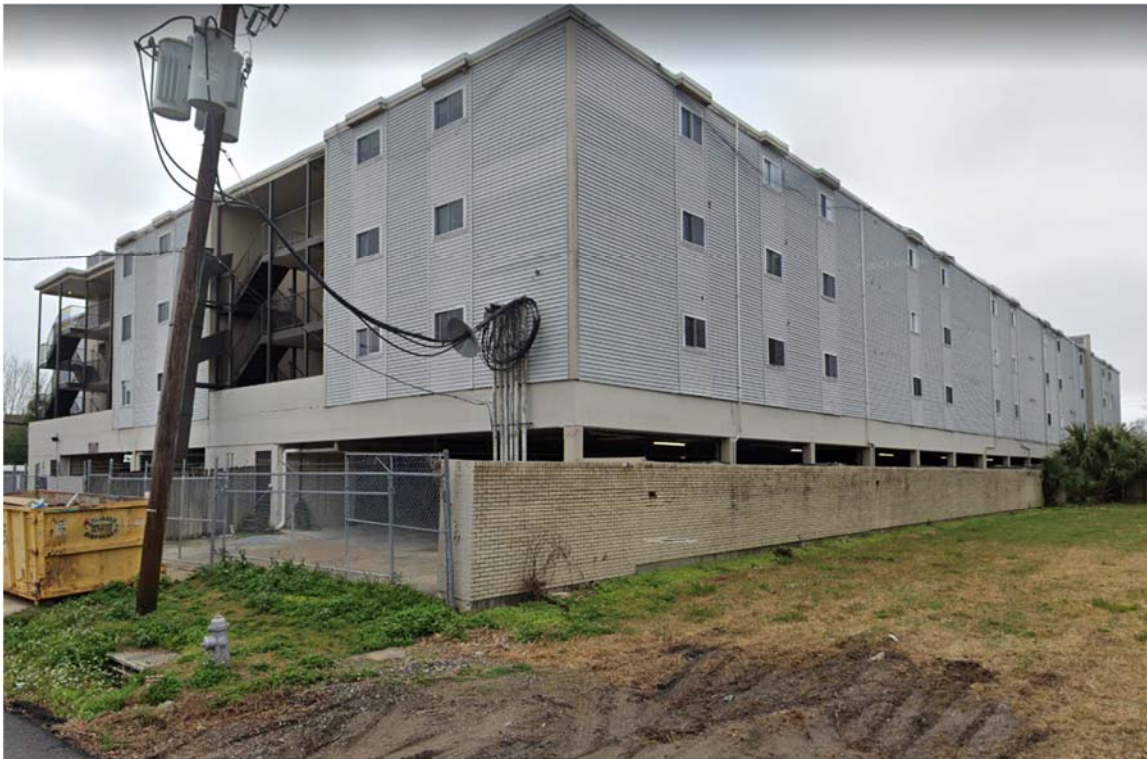
Photograph 10 - Southeast corner and east side of building
