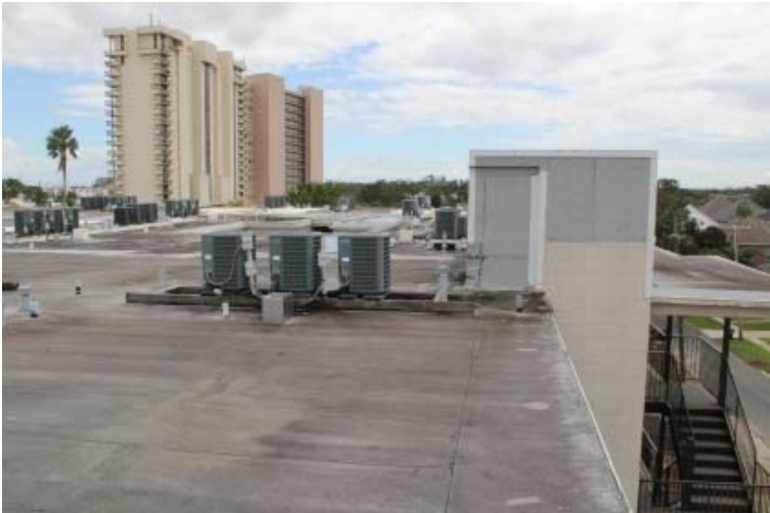
Photograph 26 - Rooftop from southwest corner – Looking east
